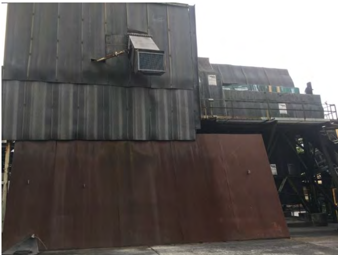
Plate 4.7 Noise mitigation cladding on CHPP
